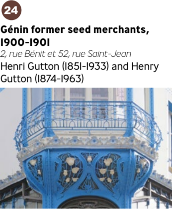
The uniqueness of this building lies in the decision taken by Henri Gutton and his nephew Henry Gutton to leave the riveted steel structure entirely visible. Jacques Gruber created the stained glass windows decorated with wisteria and poppies. This motif can be found on the oriel's ironwork of the and on the ceramic frieze.
