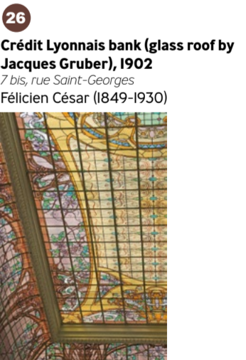
The Crédit Lyonnais branch reveals style of Félicien César, with a classical façade, a metal structure borrowed from the Construction industrial buildings and the use of artists from the Nancy School. The use of a metal framework to support an immense glass ceiling. The stained glass window, decorated with clematis the ticket office is the work of Jacques Gruber.
