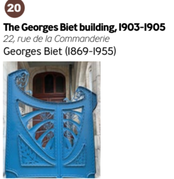
After working in his father's agency, Georges Biet decided to build a building to house his offices and residence. He opted for the use of modern materials: reinforced concrete for the ground floor slab, steel beams for the upper floors, and riveted steel for the structure. The gate combines riveted steel profiles with wrought iron decorative elements.
