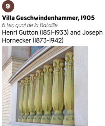
The villa is distinguished by the decorative elements on the façade by the ceramists Gentil and Bourdet, with balcony balustrades in flamed sandstone, polychrome brick arches, and mosaics framing the windows.
