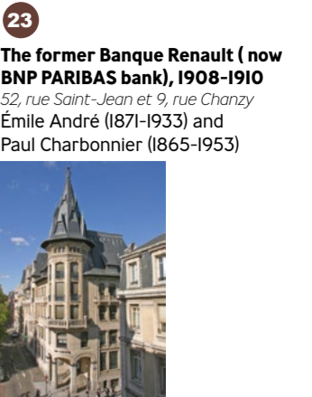
The project to modernise Renault bank is the first major in Nancy to use a reinforced concrete structure and steel structure. This choice enabled rapid construction with large spans, just like the monumental tower-porch forming the corner. The pillars, decorated with ginkgo leaves, mark the entrance to the building.
