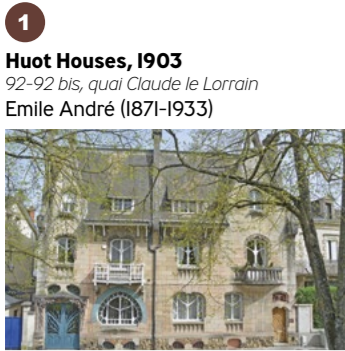
These iconic houses with false symmetry feature a façade whose verticality is accentuated by medieval-inspired gabled dormers. The use of various shapes and materials contributes to the architectural harmony, incorporating sculpted motifs of seaweed, pine cones, and flowers...
