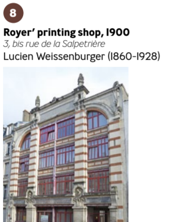
The printing works of Jules Royer is a fine example of Art nouveau industrial architecture, where brick and stone materials are combined with riveted steel to provide multiple levels of workshop space and open the façade with large bay windows. The panels sculpted by Ernest Bussière evoke the work of the printing industry.
